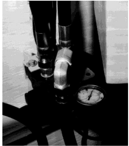
MAIN HYDRAULIC VALVE
